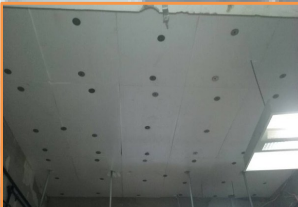
SBI, Thermacol Undertaken Insulation Vashi, Mumbai
